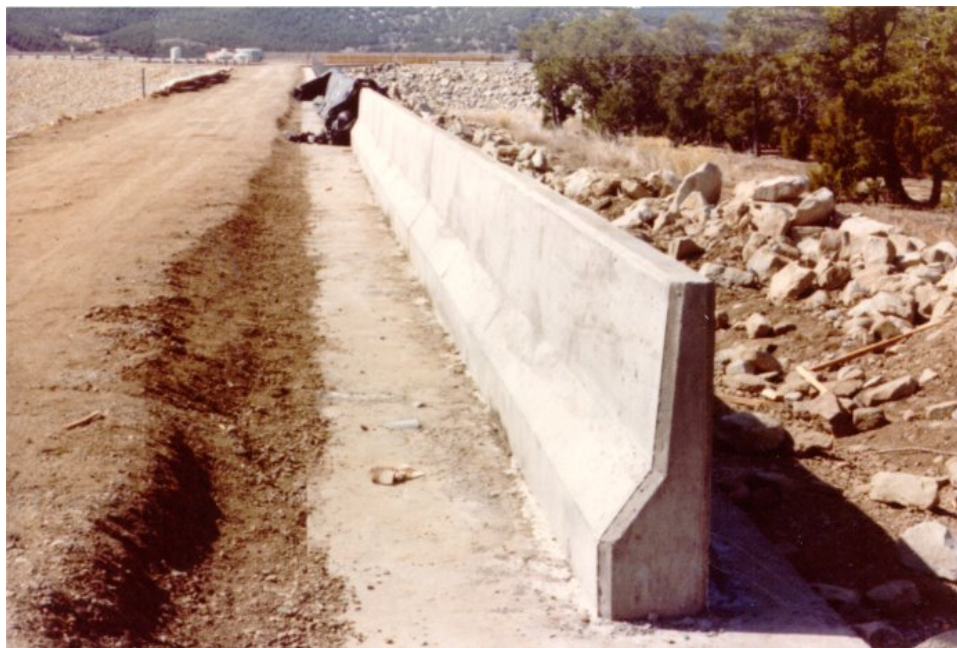
Figure F-2. Example 2: a conventional parapet wall
